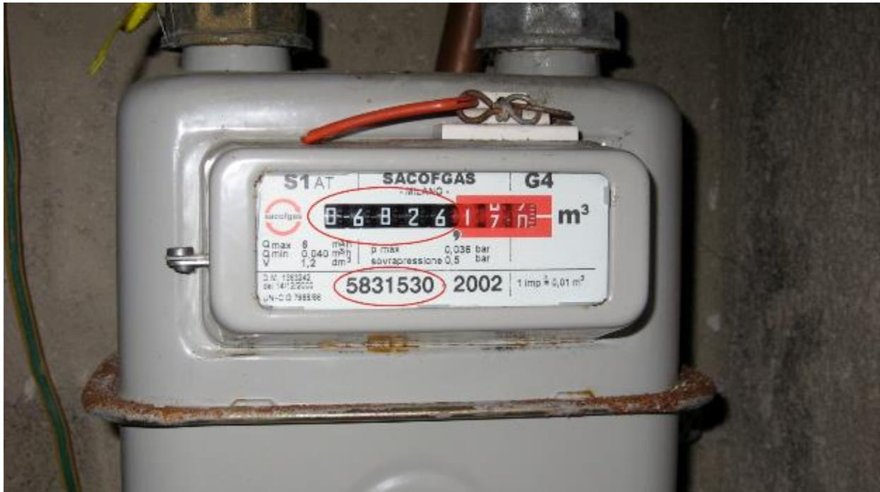
The rotary digits in black show your current gas meter reading. The red digits are less than 1 cubic meter and are not needed when we request a gas reading/to do estimations.
